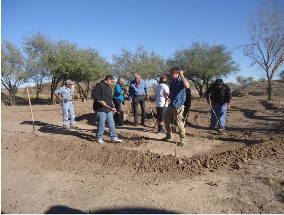
Rain harvesting garden building with Clifford Pablo, TOCC
